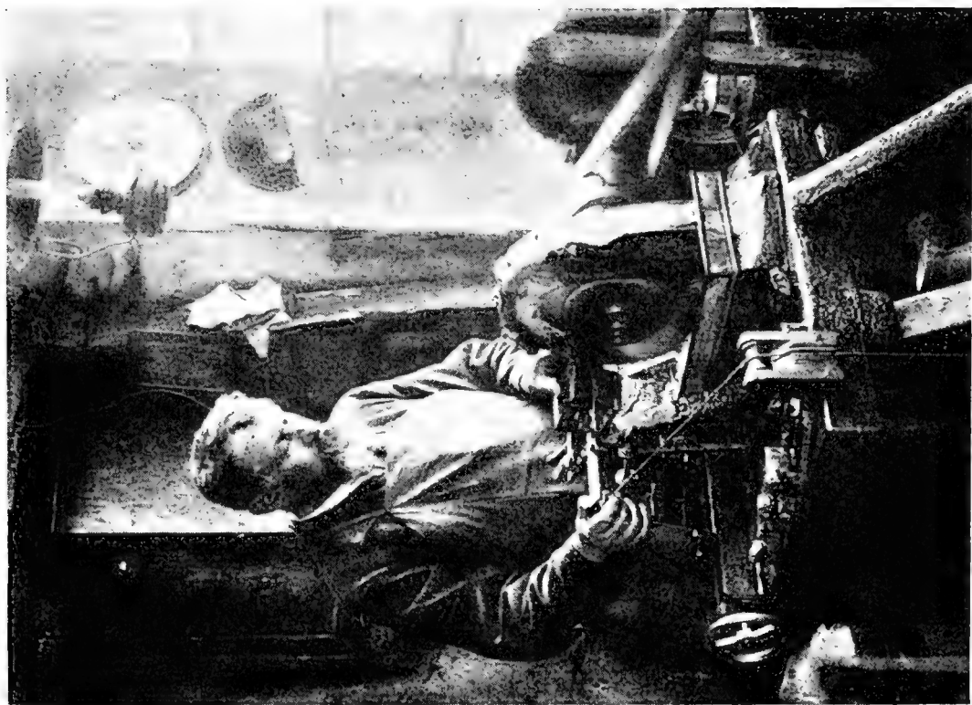
FIG. 30.—Oberstein. Slicing gems with diamond saw.
